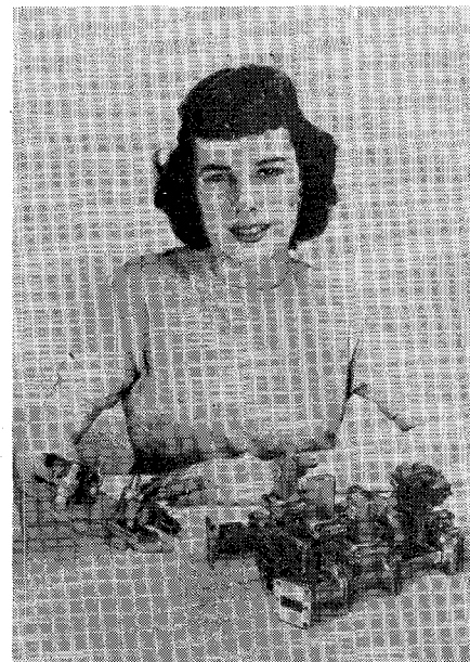
Fig. 4. This photograph was on the cover page of the Tri-plate Manual published in 1956 and shows the comparison of a Tri-plate circuit with its waveguide equivalent. (Photo courtesy of Sanders Associates.)
